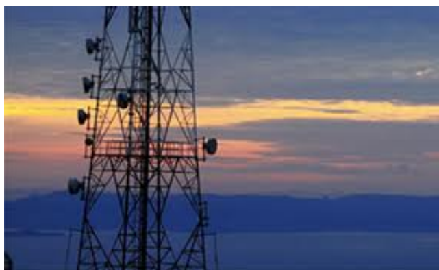
Image I. Microwave Towers Source: Google
